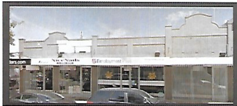
2019 81-85 Pier Street an extension & facsimile of the early frontage remains
